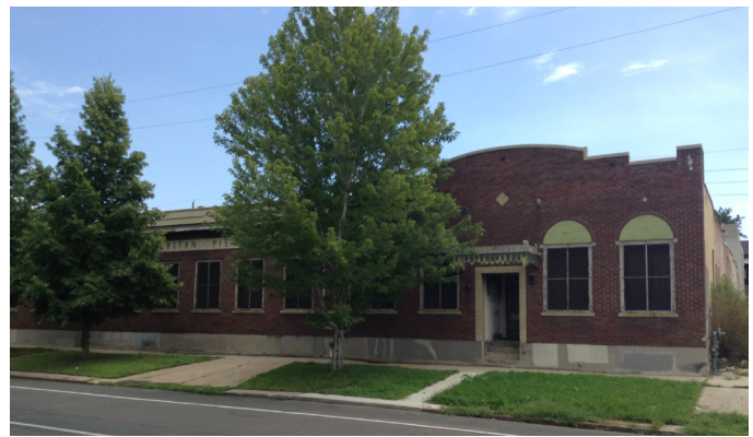
5. Typical early 20th-century commercial development within the district, featuring brick construction and raised parapet hiding a flat roof.
