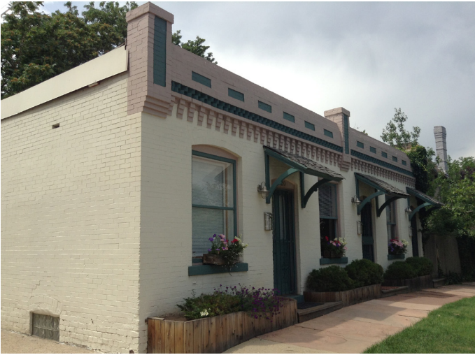
10. One-story multi-family Italianate dwelling facing onto a side street. Note the building mass aligns with the sidewalk, the decorative cornice, the segmental arched window and covered stoop entries.
