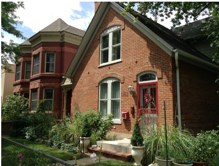
1. Streetscape within Curtis Park with eclectic architecture that characterizes the district. Note the simplified Queen Anne cottage in the foreground with orange brick façade in contrast with the elaborate, large Italianate duplex structure in the background with brick façade, stone stringcourses, window headers and sills.
