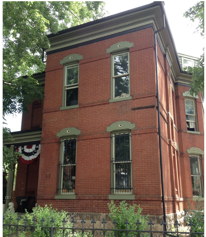
7. Typical brick Italianate structure within the district. Note the decorative cornice, the tall narrow windows with elaborate stone window headers and sills, the low pitched roof, rectangular projecting forward bay and stone foundation.
