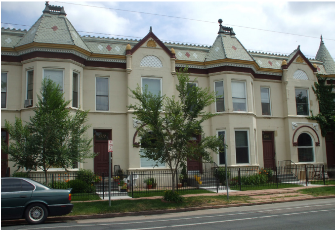
4. Multi-family Victorian eclectic dwelling fronting onto a primary street. Note this repeating projecting towers, the arched windows on the first floor with decorative headers, the transoms above the single entry door, and the decorative pattern roof.
