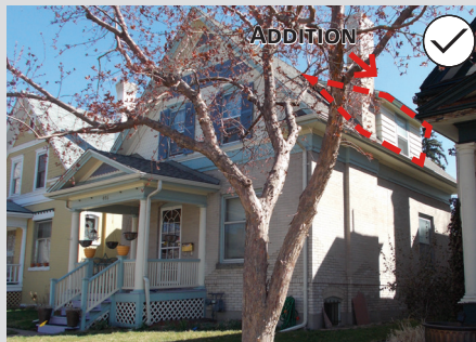
65. An appropriate side shed dormer addition, located behind the chimney. See "Dormer Location" on page <?> for more information.
