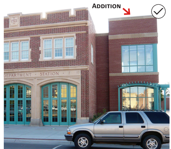
69. Differentiate an addition from the original structure with an offset of at least four inches and/or with a change in material or size.
