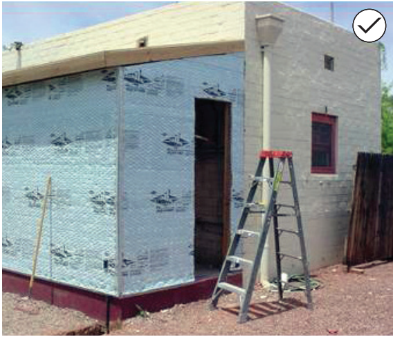
70. Do not damage historic building fabric or obscure key character-defining features of the primary structure when building an addition.
