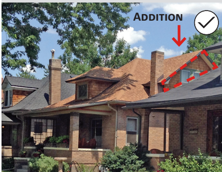
64. Appropriate side-gabled dormer addition that has minimal impact on adjacent contributing properties.
