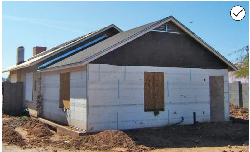
71. Use a roof form that is consistent with the original structure's roof form and those of structures in the surrounding historic context. A "nested" gabled addition is being added to the bungalow house illustrated above. There is no street visibility and the roof form matches the historic house.
