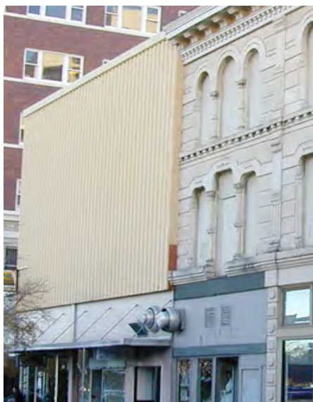
8. Remove later covering materials that have not achieved historic significance. The covering illustrated at left was removed to reveal the underlying historic materials (right).
