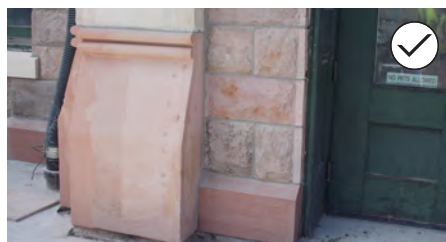
30. If necessary, repair a foundation wall using new material that is similar in character to the original. The foundation illustrated in the top image was patched with a consolidant that was tinted to match the existing pink sandstone, as illustrated below.
