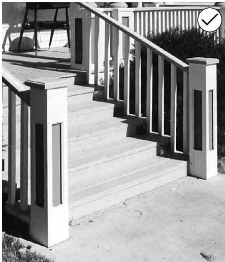
39. Maintain and repair historic porch and stoop components, finishes and details. For example, this deteriorated porch railing illustrated at left has been restored to its original condition, as illustrated at right.
