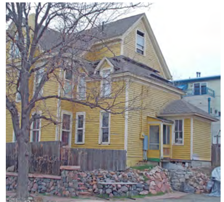
2. Contributing addition to a historic structure.
