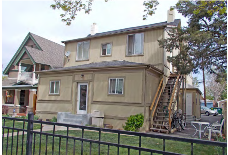
4. Non-contributing house in a historic district
