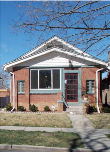
3. Non-contributing porch infill/enclosure in a historic district
