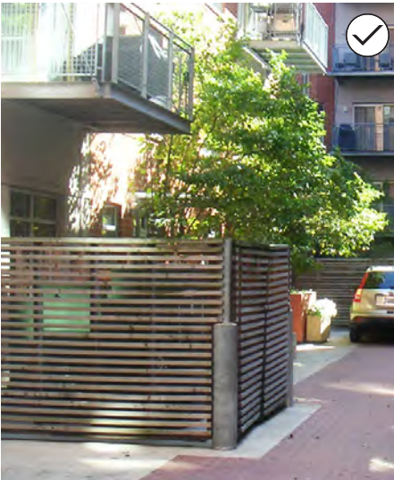
123. Screen ground-mounted mechanical equipment.
