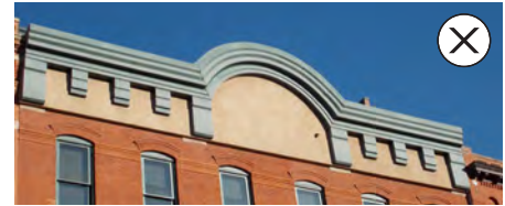
25. Avoid removing or covering original roof materials and features that are in good condition. The original brick parapet on the building illustrated above is covered with a stucco and wood replacement that does not match the original.
